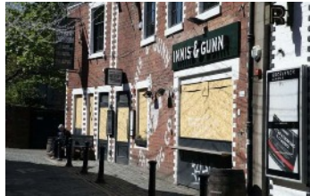
A boarded up pub in Glasgow
